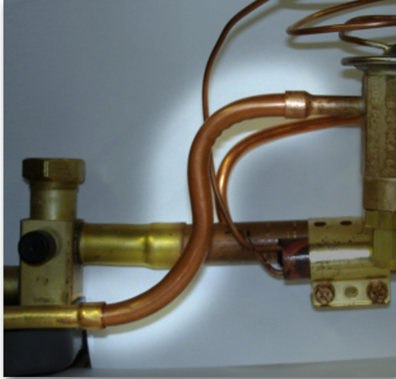
Figure - 1. Bend pipe to "S" shape.
