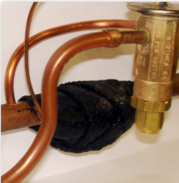
Figure - 7. Insulate the Sensor bulb as well as both refrigerant lines.
